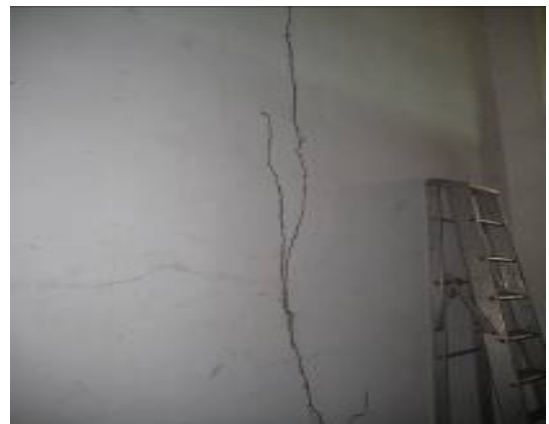
A termite path in the warehouse
