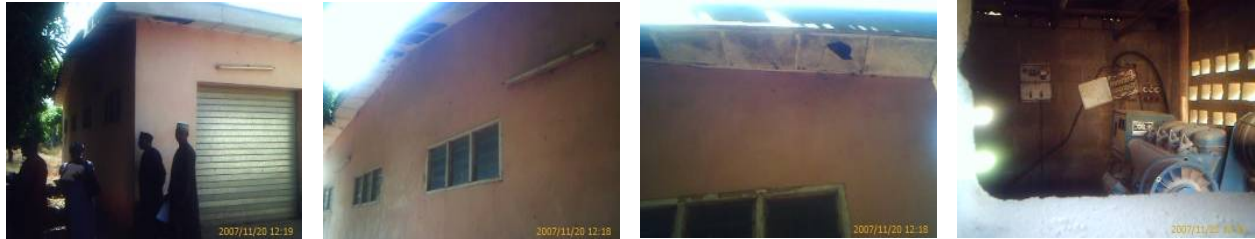
Kaduna warehouse as seen from the outside
